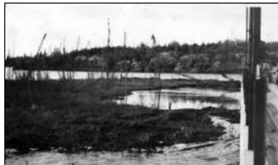
Floating island being pulled in-shore to be broken up and shot over the dam outlet outside the danger point to the power plant.
