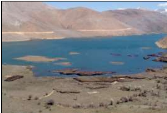
Abdulharap, (Çat Dam), Adiyaman
