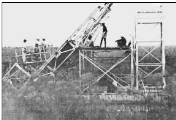
On trial, 1953. The cutters have been lowered.
