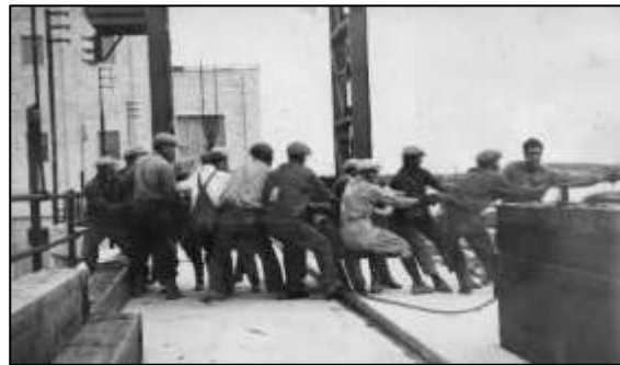
Floating island being pulled in-shore to be broken up and shot over the dam outlet outside the danger point to the power plant.
