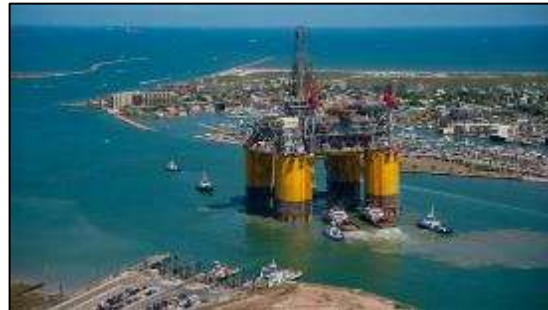
Olympus, a tension leg platform production facility, will be moored from each corner.
