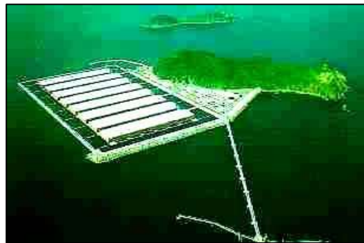
Shirashima Floating Oil Storage, Fukuoka City, 7 barges, 397 by 82 by 25.1 meters, 5.6 million cubic meters, built in 1996
