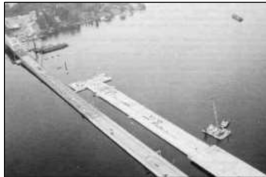
Homer M. Hadley Bridge in construction
