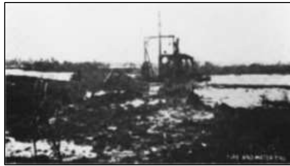
Rake being returned to position and rake pulling a portion of an island ashore
