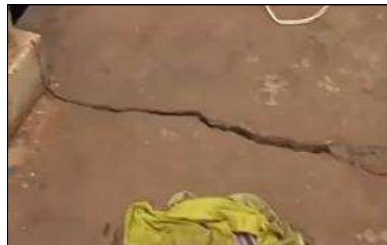
Photos from 2010, the one to the right, evidence of under-reinforcement.
