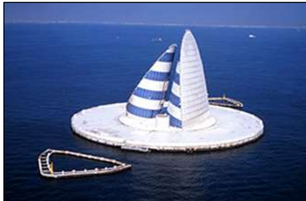
Ventilation shaft for the Tokyo Aqua-Tunnel expressway connecting Kawasaki and Kisarazu
