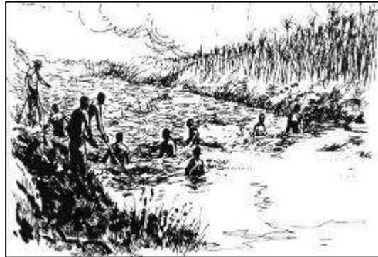
A few days later, a secondary obstruction of matted roots, etc., rises to the surface and must be removed.
