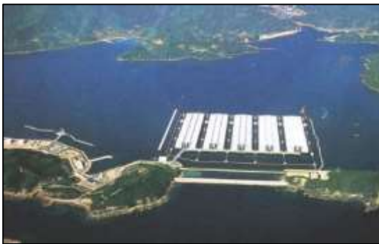
Kamigoto Floating Oil Storage, Nagasaki, 5 barges, 390 by 97 by 27.6 meters, 4.4 million cubic meters, built in 1988
