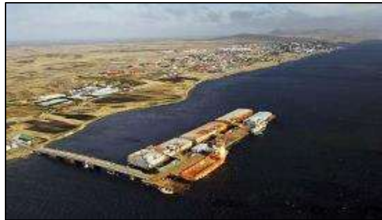
A floating pier for drilling vessels, Falkland Islands
