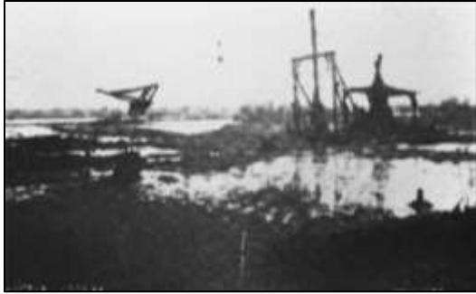
Rake being returned to position and rake pulling a portion of an island ashore
