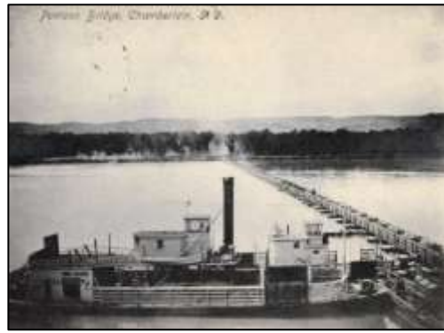
Chamberlain, South Dakota. 366 feet, constructed in 1905, developed leaks in 1918, and replaced by girders.
