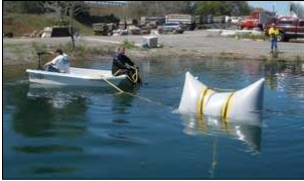
Towing into position
