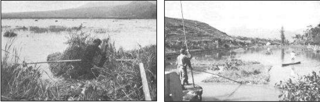
Sawing an island of aquatic plants in Rawa Pening Lake and poling it to the spillway
